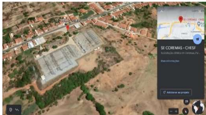
Figure 2: Location of the Coremas Substation – CHESF. Source: Google Earth (2023)
